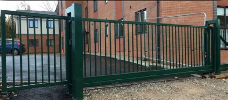
Metal Sliding Gate Installation
